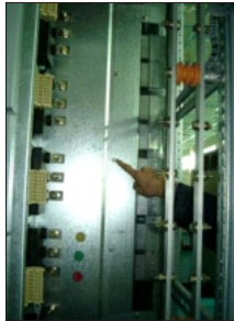
Remove the transparent cover for the linkage busbar
