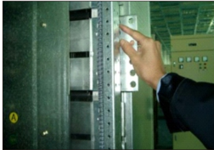
Install the linkage busbar in each cubicle
